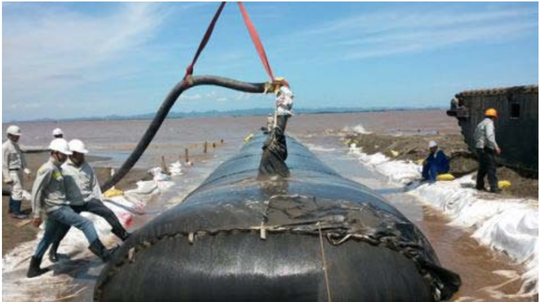
Figure 2: Geo-tube filling using drag pump
